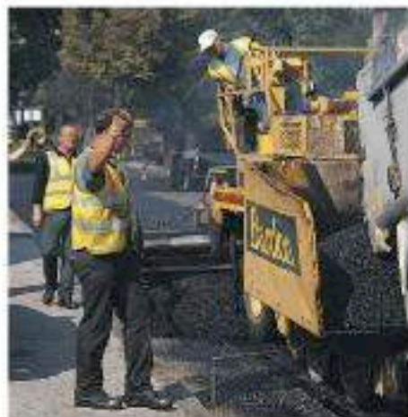
Figure 20.8 Bitumen is used in road construction.
