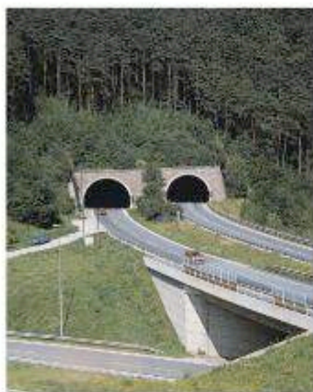
Figure 6.25 Traffic passes easily through a road tunnel under a mountain.
