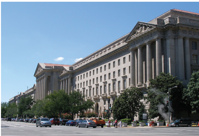
FIGURE 12.5 The office building for the U.S. Environmental Protection Agency, Washington, DC.
